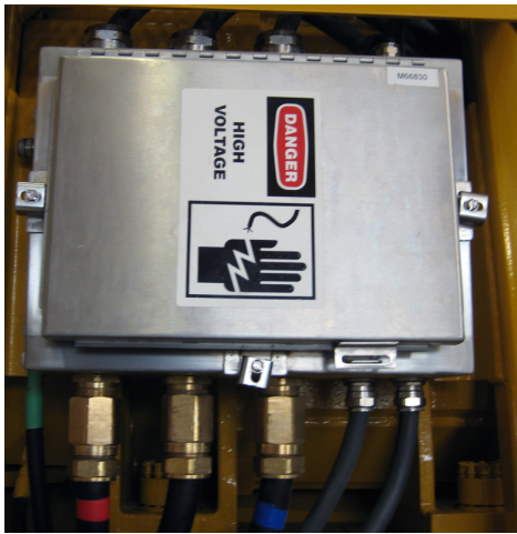
Figure 1: Enclosure DT13672 and Replacement Gasket DT13672-1
